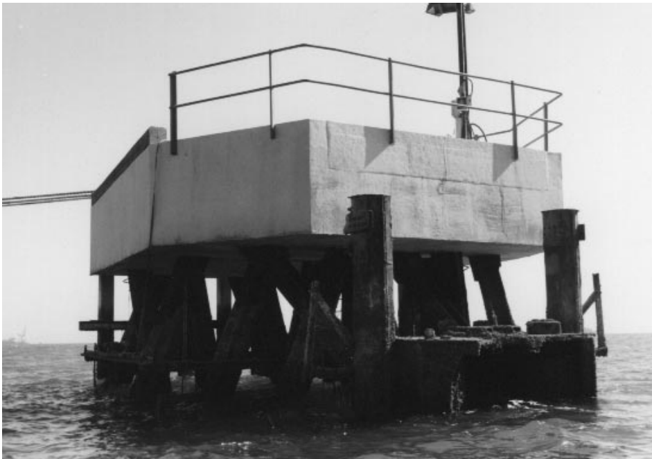
Figure 5: Concrete structure one and a half year after repair (1999)
