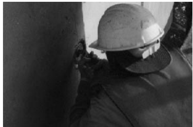
Figure 7: Fitting of the zinc contacts
