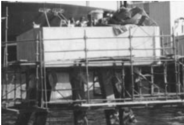
Figure 8: Concrete structure after repair
